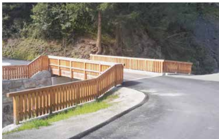
Recently, the two bridges over the Bangartbach and the Hobarbach in the Geiselhöfe area of Tux-Vorderlanersbach were replaced.
